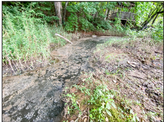
This unnamed creek was contaminated with sewage spillover after a private lift station failed in the Hawks Harbor area of Lake Chatuge. The leak was contained July 3. Photo/Facebook
